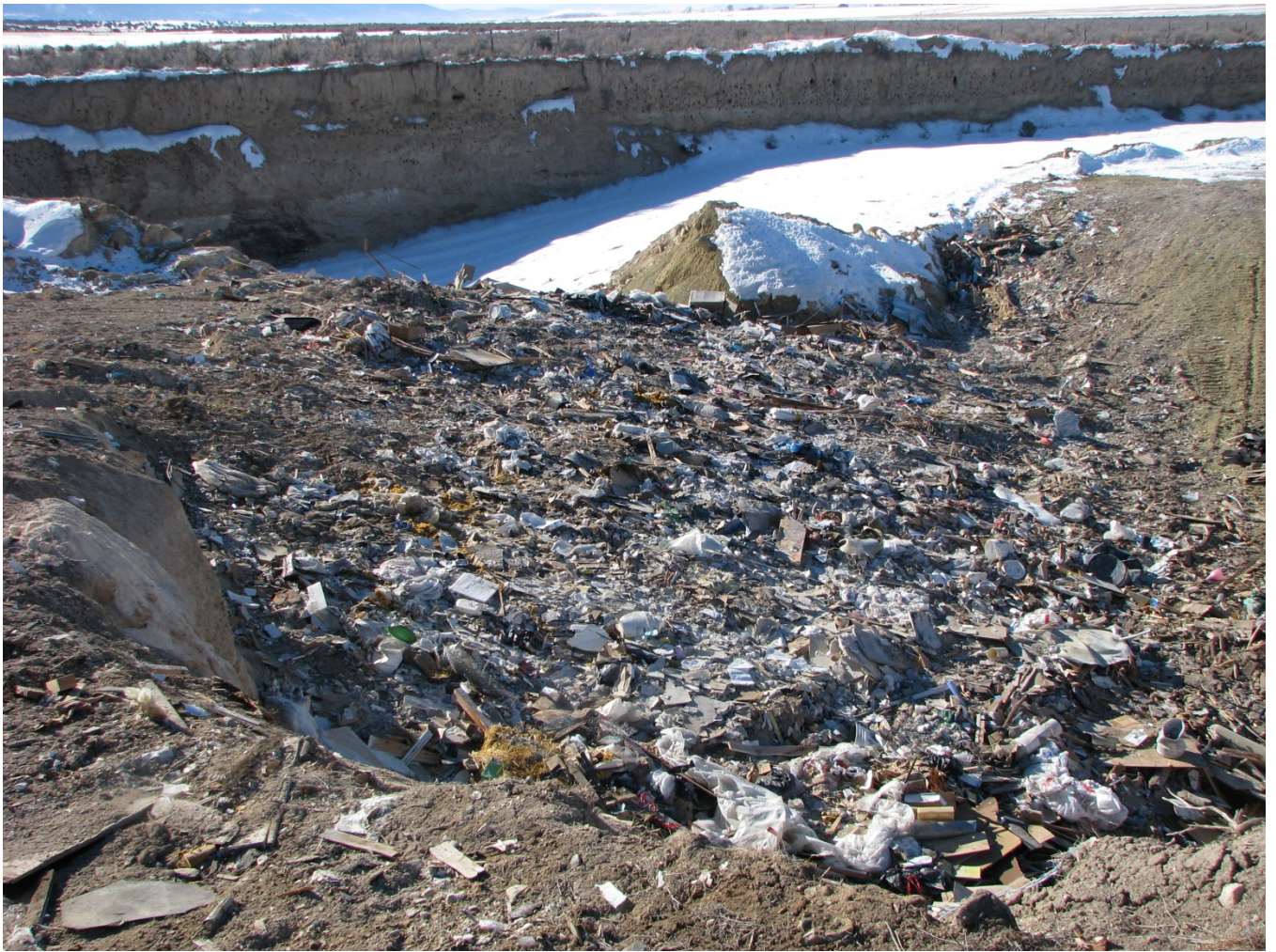
The working face of the landfill
